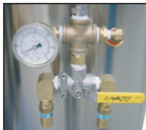
Dual Relief Valve Assembly
